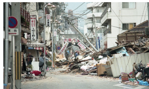
[神戸市灘区被災状況]
